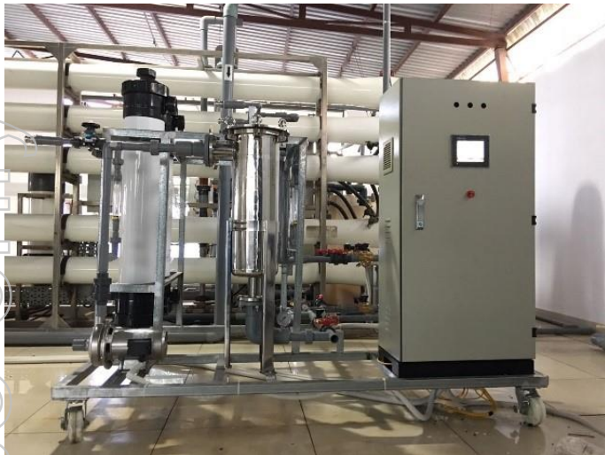
Pictures: Pilot water treatment systems for filtration of water from nearby Mekong River in Duc Hoa, Long An Province, Vietnam
