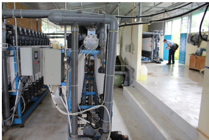
Water treatment plant in Nghe An province, Vietnam, sold by De.mem – hollow fibre membrane water treatment systems and control panel
