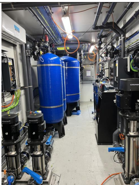
Image 2) De.mem Containerized Membrane Based Water Treatment Plant
